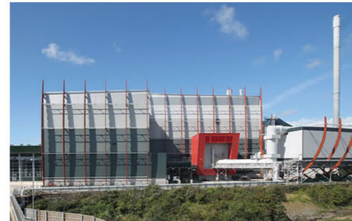
Example EfW facility already constructed using the proposed EfW technology provider
